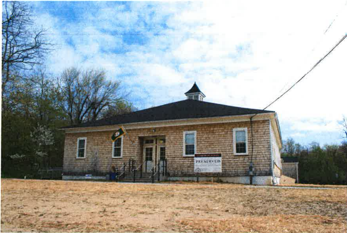
The Old Clarksburg School Was Renovated to Become the New Millstone Township Municipal Building
